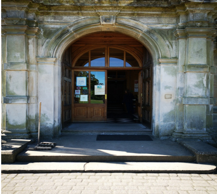
View of our main entrance from Callendar Park
